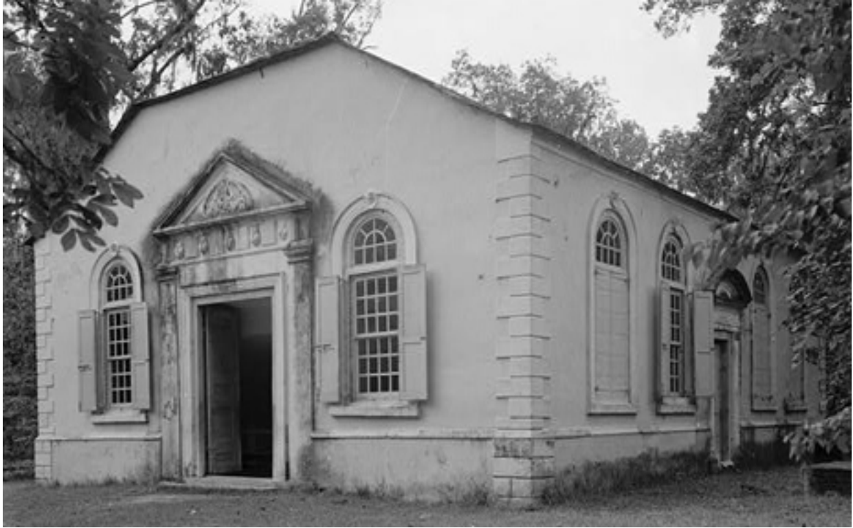
St. James's Parish Church, Goose Creek (1706-1719; HABS)
