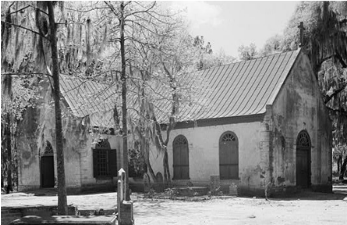
St. Andrew's Parish Church (1706, 1723; HABS)
